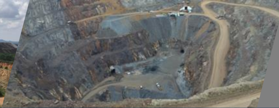
Transitioned to underground with forced portals $0.5m
