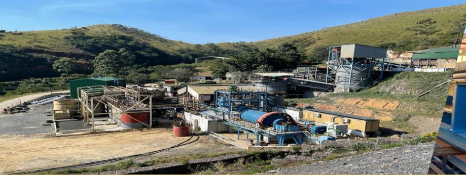
Jaw crusher, cone crusher, mill and then float.
